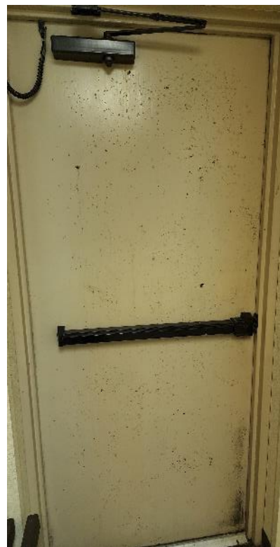
Picture: Rusted Parish Center back door
