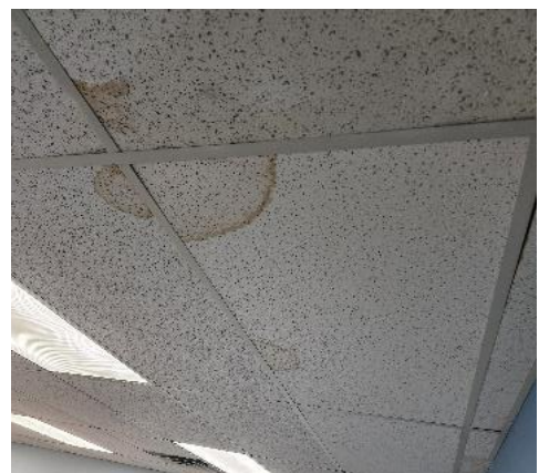
Picture: Roof leak over meeting room 211
