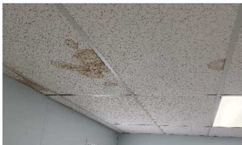
Picture: Roof leak over meeting room 211
